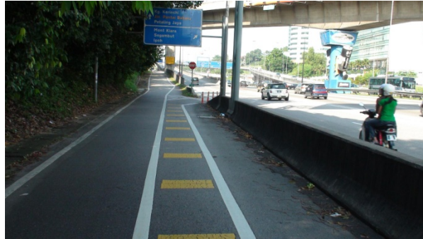
Fig.1. Road Surface after Pavement Marking Installation, F02 Highway, Malaysia
