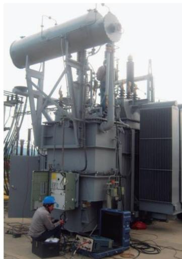
Figure 4. Typical power transformer 115 / 13.8 kV
